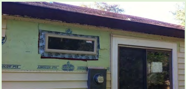
IN THESE PICTURES, A TAN WESTVIEW VINYL WINDOW WAS INSTALLED IN THE MASTER BATH OF A HURON MODEL HOME
